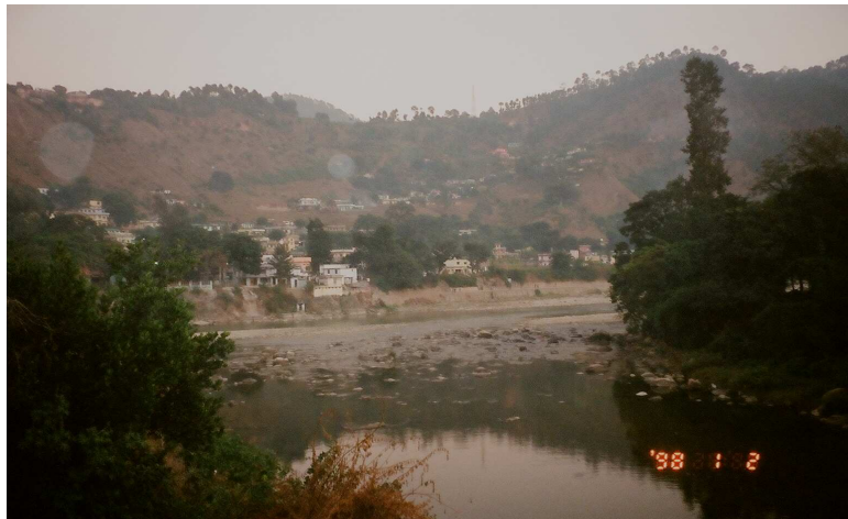
Photo 2.1: Drainage view of Bageshwar
